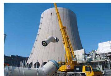
The IPB, a high current connection between generators and step up transformers, is a key component to transfer electricity to the power grid and also for unit auxiliary supply within a power plant. The IPB design has to fulfill all requirements relating to operational reliability and safety.
